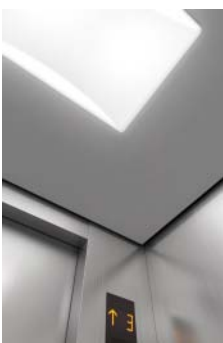
Ceiling: Painted steel sheet (Y033) with a milky white resin lighting cover Lighting: Central lighting
